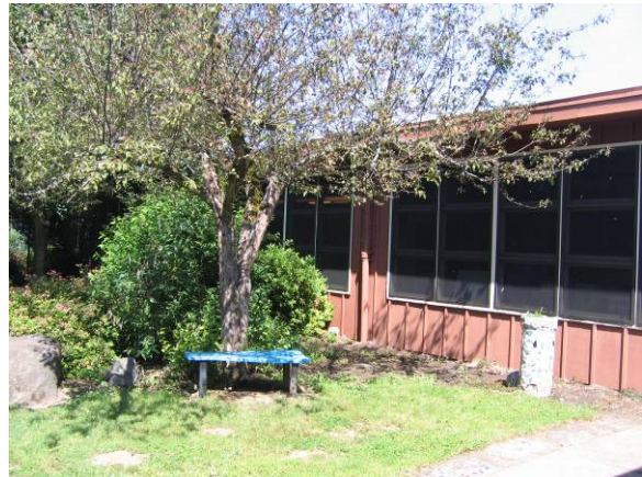
Interior courtyard and south elevation windows
