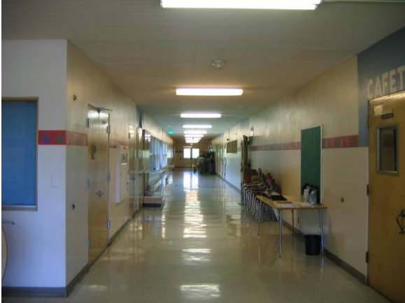
Corridor facing north
