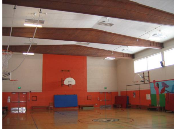
Gymnasium facing north
